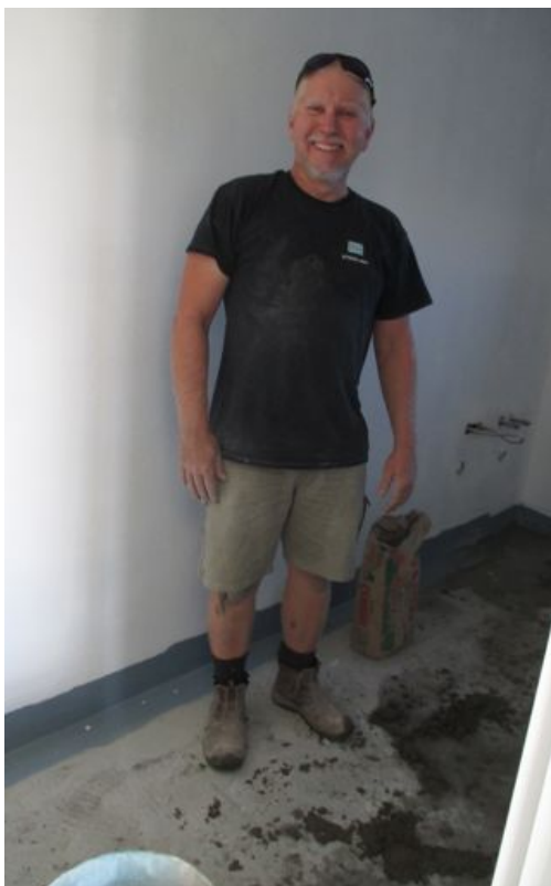
Michael, the tiler, cementing the floor in the Amenity Block
