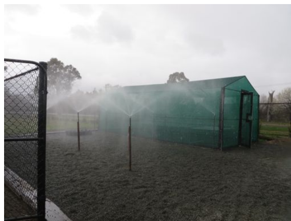
Testing the irrigation system
